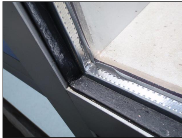
Figure 7 An Example of Primary Sealant Infringement
